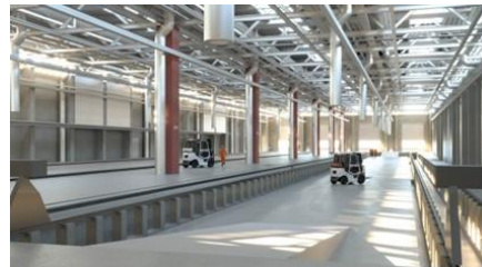
Workshop for electric trains DSB (Danish State Railways)
