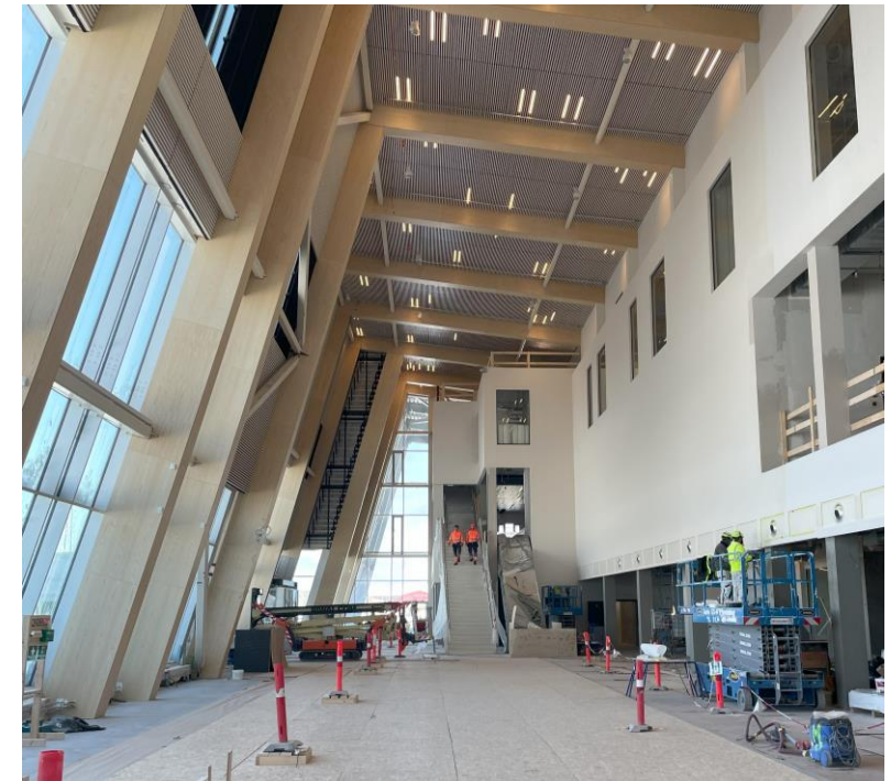
Airport in Nuuk
